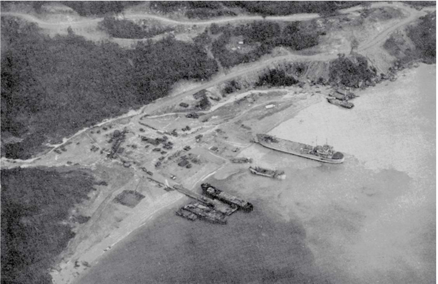
Barely three months after engineers of 39th Combat Engineer Battalion began transforming the area from soft sand and tangled underbrush, Port Lane is in operation for 1st Logistical Command support operations.
